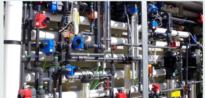
* Pilot plant view
