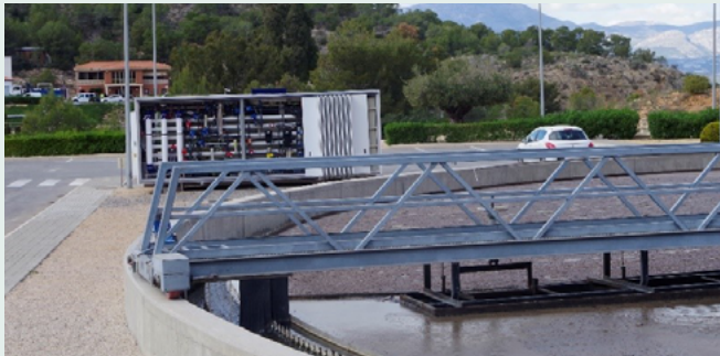
* Location of the pilot plant within the Benidorm WWTP
