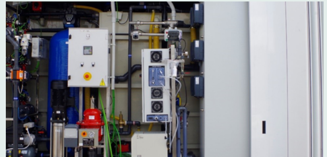
* Pilot plant view
